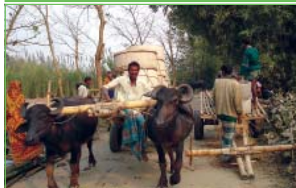
Figure 36: Community working together for installation of sanitary latrine, Kurigram, Bangladesh
